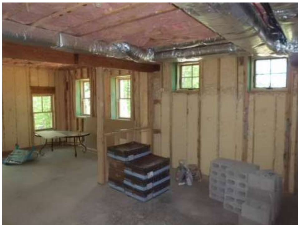
Figure E- 8: Walls with Closed Cell Spray Foam Insulation
