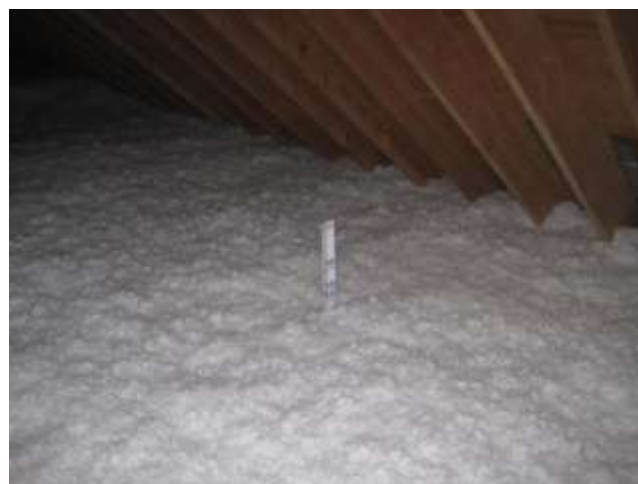
Figure D-6: Grade I Blown Fiberglass—Attic
