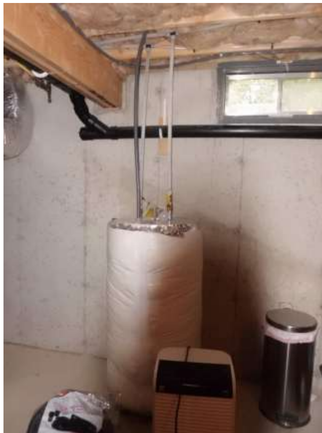
Figure E-15: Insulated Indirect Water Heater
