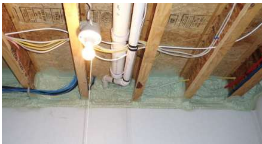
Figure E-7: Rim Joist Insulated with Spray Foam
