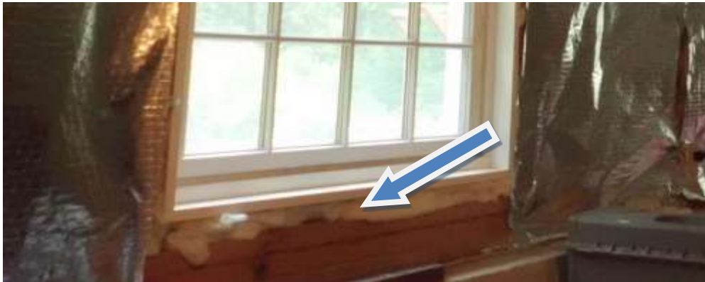
Figure E-12: Fiberglass as Ineffective Air Sealing
