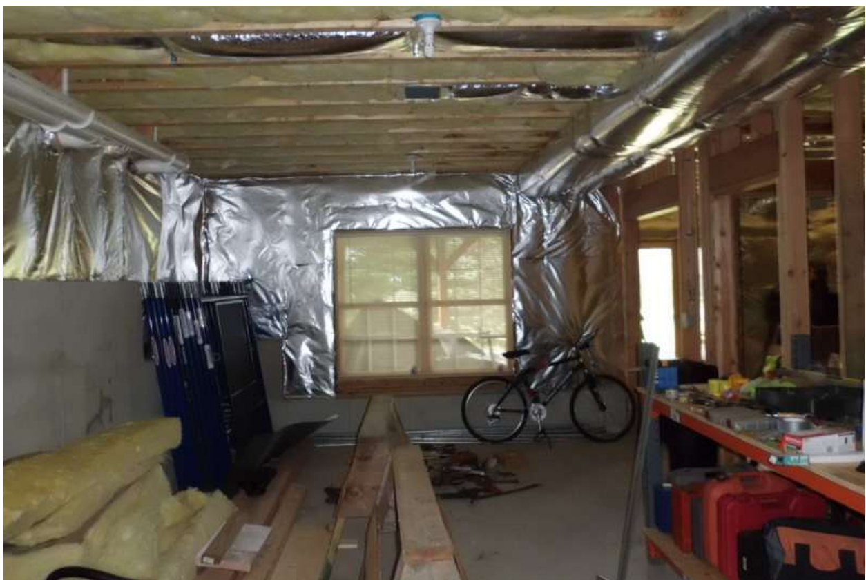
Figure E-2: Insulated Walkout Basement Walls
