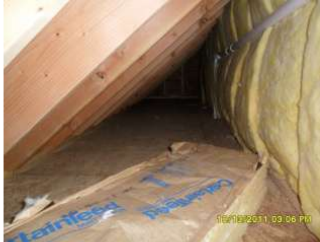
Figure D-3: Grade III Fiberglass Batts—Attic Kneewalls
