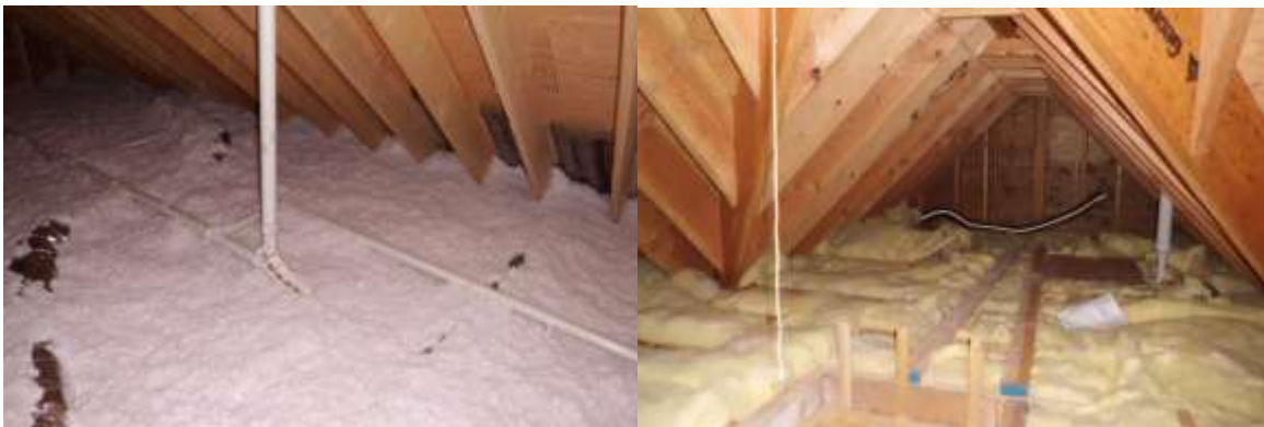
Figure 1-2: Example of Grade I and Grade III Attic Insulation Installation
