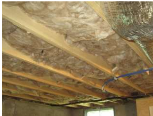
Figure D-4: Grade II Fiberglass Batts—Frame Floor
