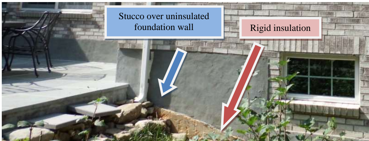
Figure E-1: Foundation Wall Rigid Insulation
