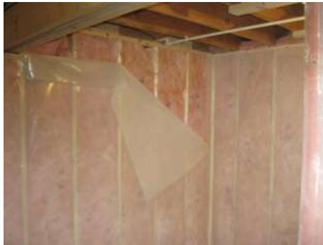
Figure D-2: Grade II Fiberglass Batts—Basement Walls
