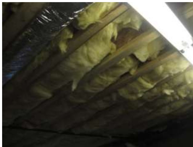
Figure D-5: Grade III Fiberglass Batts—Frame Floor
