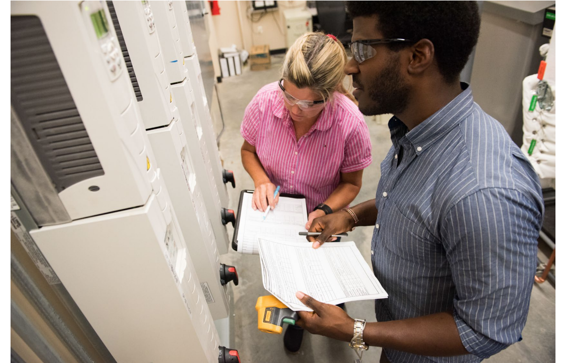
Building research engineers develop and demonstrate advanced technologies and methods for evaluating building performance. Source: Pacific Northwest National Laboratory, 2017.
